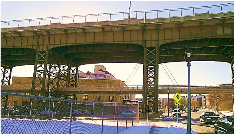
The Holton Viaduct and Marsupial Bridge
