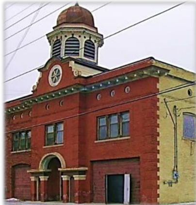
Old firehouse and village hall buildings on 35 th St. south of Villard
