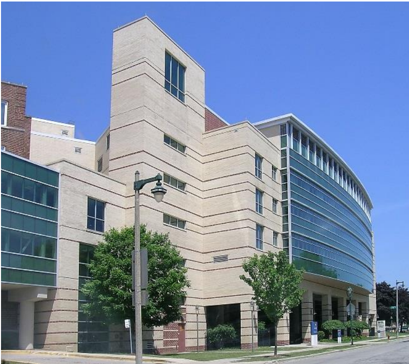
Ascension SE Wisconsin Hospital—St. Joseph's Campus
