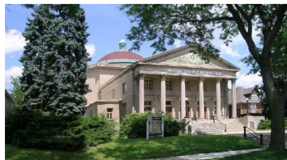
St. Luke Emanuel Baptist Church at 27 th & W. Highland Blvd.
